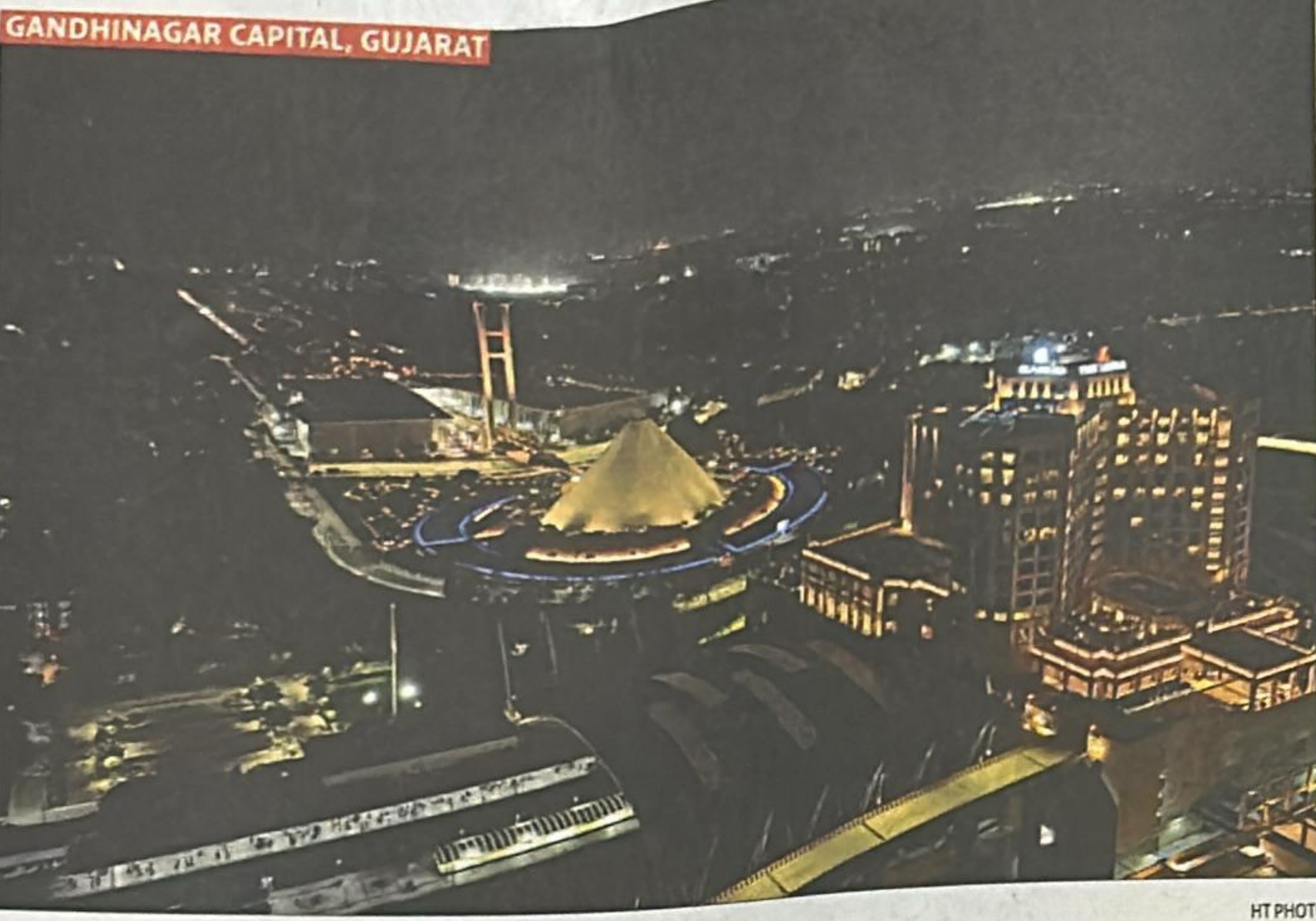
The Gandhinagar Capital railway station has a hotel atop.
